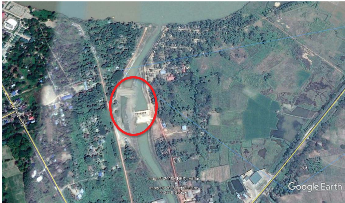
Figure 25 Barrages at Mezali on the Pathein Road (16° 56' 38.10" N 95° 47' 52.34" E) are an example of blockages preventing connectivity between floodplains and rivers.
