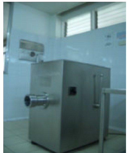
Fig. 472: Hygienically good finishing of premises. Wall tiles and wall windows 2 meters high, for easy cleaning.
