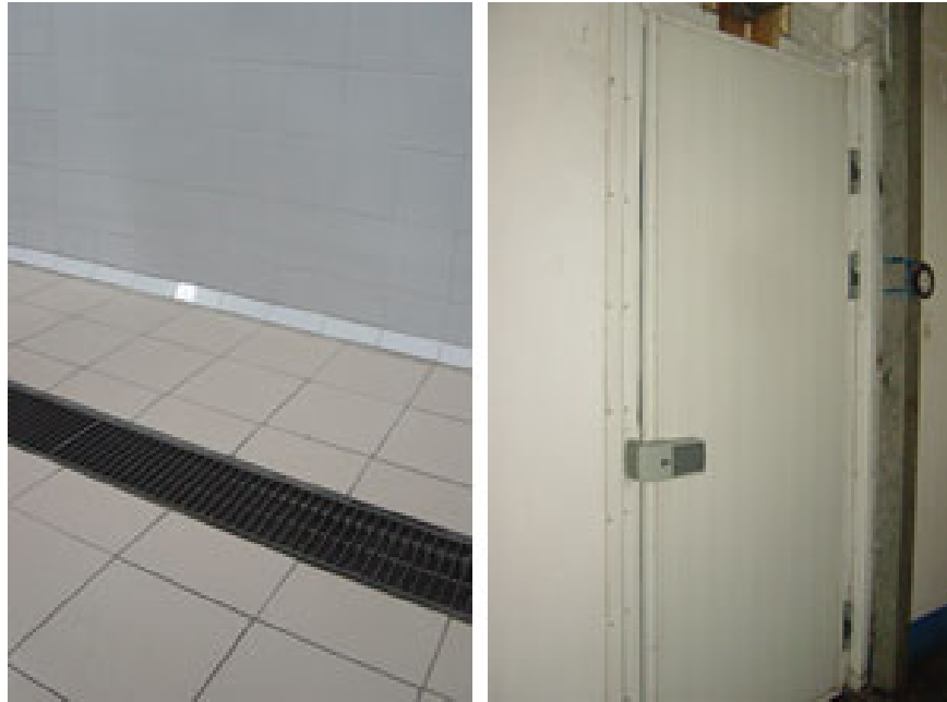
Fig. 473: Hygienically good finishing of premises. Easy to clean surfaces, left floor with drain and wall with coved junction, right plastic door for refrigerated room.
