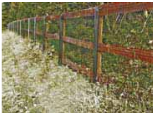
Game preserve fences can have various construction appearance
