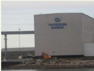
The horizontal structure which can be seen on the LH side of the photo is the feeding conveyor which can deliver into the fish holds directly or into the hoppers of a road transport vehicle.
