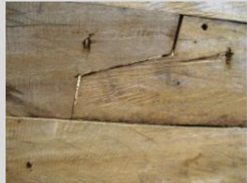
Outrigger type three. Details of the panel joints of wooden boat construction.
