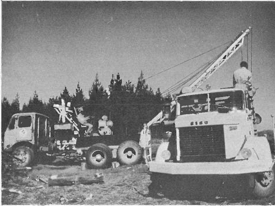
Loading logs on to a truck with a locally-manufactured truck-mounted cable-crane using a double-drum winch set from a crawler tractor. Logs were transported by a Sisu truck with trailer carrying capacity of about 17 m 3 (Forestry Commission, Erin Estate) (Photo: H. Seppänen)
