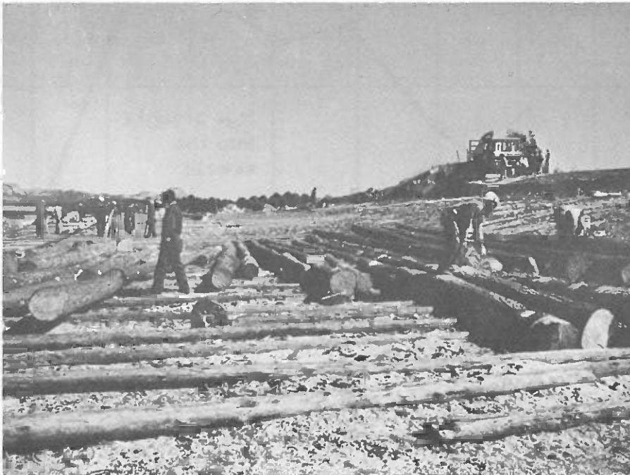
Logs crosscut at the logyard by chainsaw into short log lengths and rolled by gravity to a feed chain for the mill (Forestry Commission, Erin Estate) (Photo: H. Seppänen)
