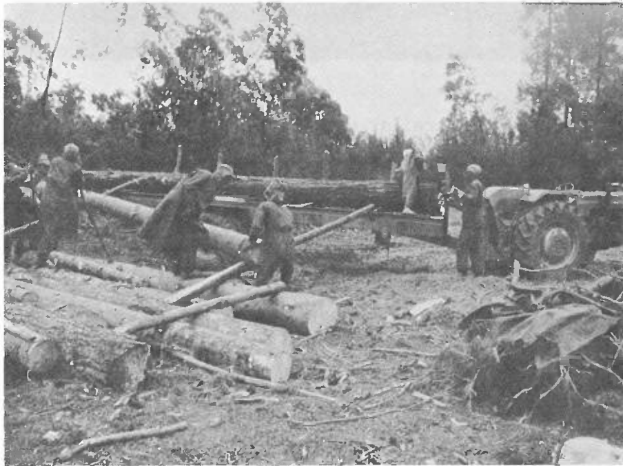
Manual loading of an agricultural tractor with trailer by an eight-man crew. Loading production was 6 m 3 /hour (Troutbeck Sawmill Ltd.) (Photo H. Seppänen)
