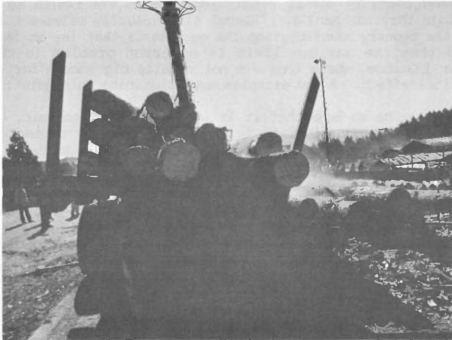
Trucks unloaded at the logyard by driving them up a slight ramp and releasing the stakes. The force of gravity helps in rolling the logs off the platform (Border Timbers Ltd.) (Photo: H. Seppänen)
