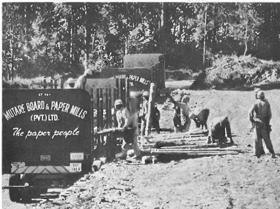
Manual loading of pulpwood on to 25-ton trailer at the intermediate landing (Mutare Board and Paper Mills) (Photo: H. Seppänen)
