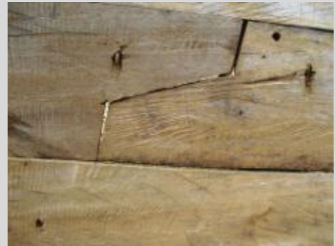
Outrigger type three. Details of the panel joints of wooden boat construction.
