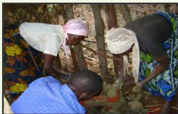
Women constructing improved stoves.
