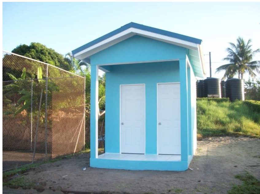
New showers constructed at Anse Ger Secondary School in Saint Lucia
