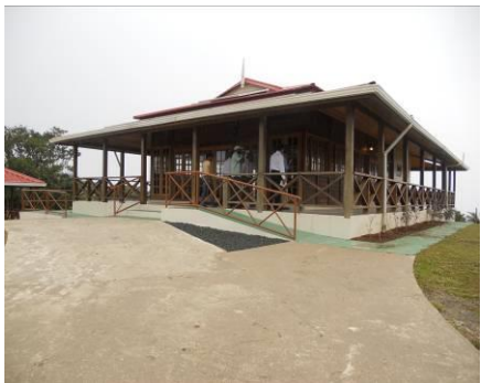
Picture 5 Large, newly constructed Visitors' Centre at the Main Ridge Forest Reserve
