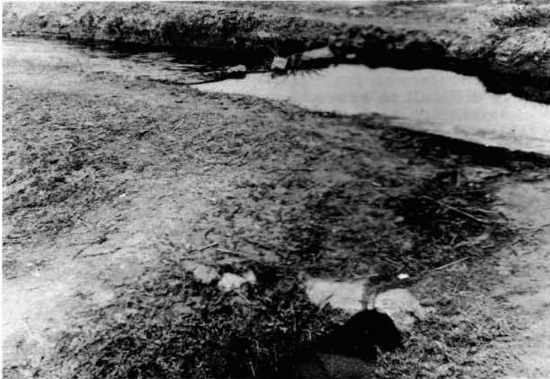
FIGURE 2-4. - Example of tampering. Brush and stone dam built by farmers across a minor irrigation canal to increase flow through a pipe outlet.
