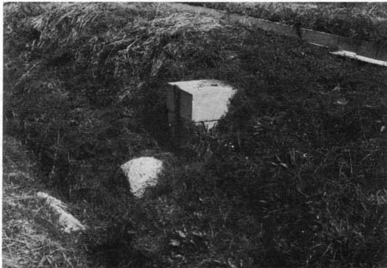
FIGURE 5-50. - Prefabricated gated outlet (Ferrara type).
