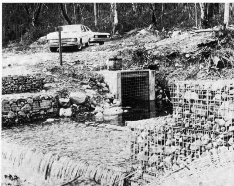
FIGURE 3-33. - Another view showing stone mesh basket construction and inlet box.
