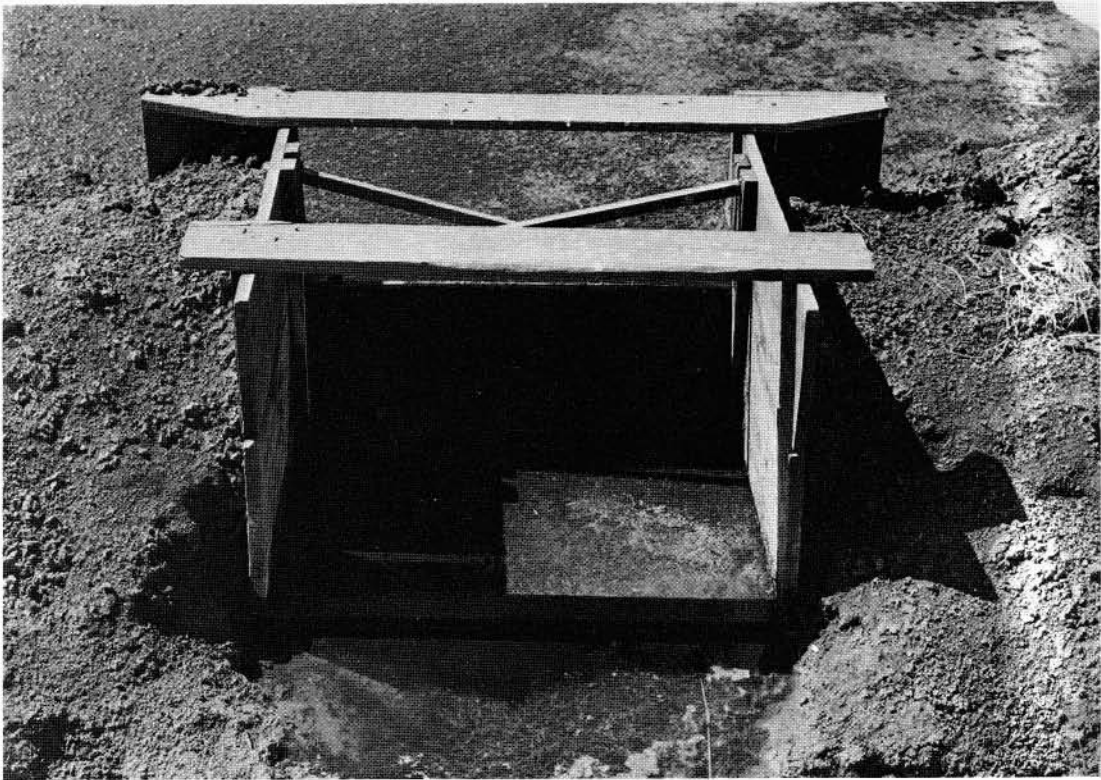
FIGURE 5-60. - Wooden outlet for basin or border irrigation.
