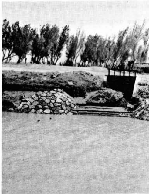
FIGURE 3-1 (a) and (b). - Silt deposition at the intake to a secondary canal.
