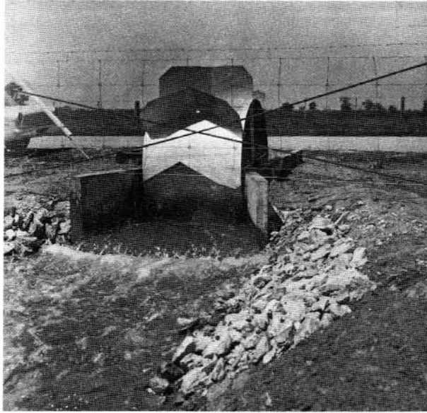
FIGURE 5-5. - Large Dethridge meter outlet in operation with free outfall.
