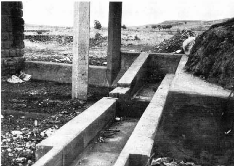
FIGURE 3-39. - Photograph of groyne intake structure (Cyprus).
