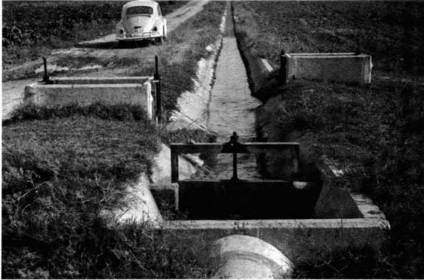
FIGURE 3-7. - Constant-head orifice farm turnouts with check-gate in foreground - East Ghor Canal Project, Jordan.
