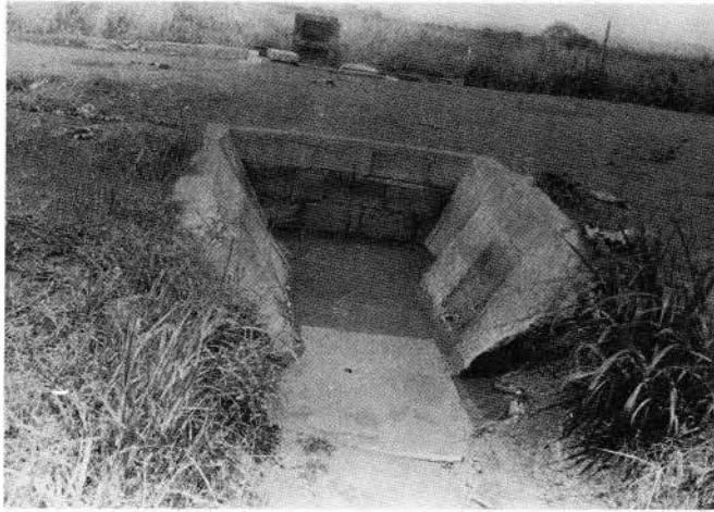
FIGURE 3-25. - Intake structure on secondary canals, outlet to tertiary canal.
