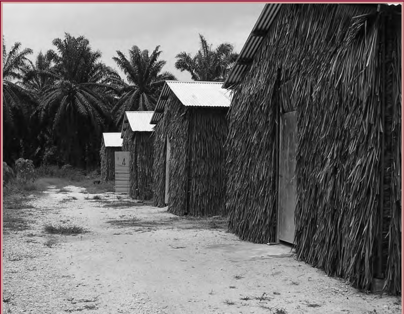
FIGURE 11 Mushroom houses with walls built from oil palm leaves (Photo by N. G. Nair)
