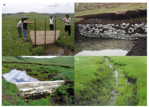
Peatland restoration. Blocking canals by a: wood plank; b: peat; c: concrete damming; and d: revegation
