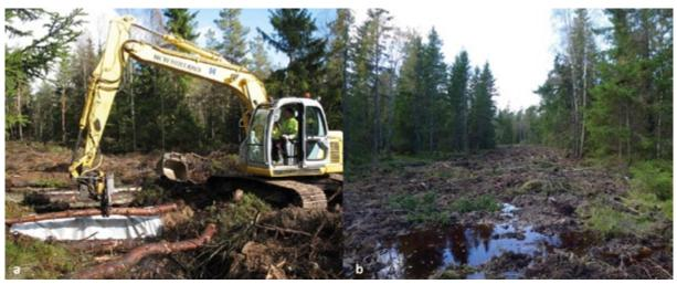
Rewetting the peatland a: Excavator building dams and filling ditches in drained fens and wet forest and b: rewetted site immediately after the completed restoration actions.
