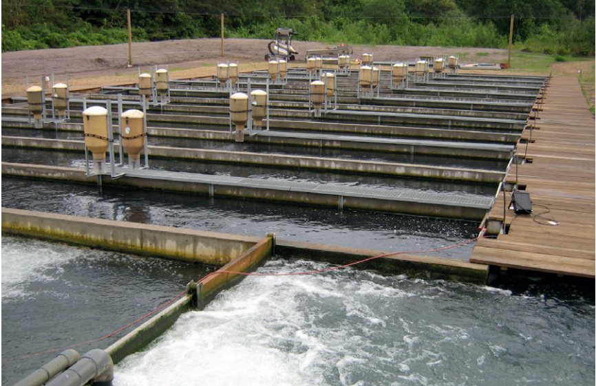
Figure 1.3 An outdoor recirculation farm.
