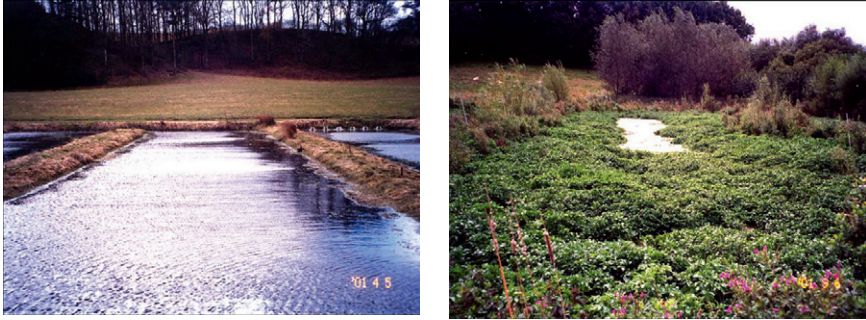
Figure 6.5 A plant lagoon placed after a recirculation trout farm in Denmark - before and after overgrowing. Source: Per Bovbjerg, DTU Aqua.
