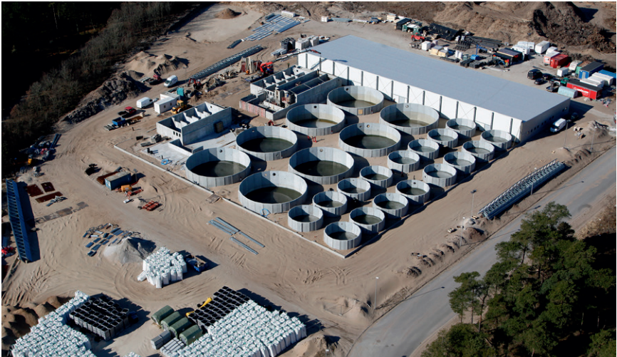
Figure 8.5 A 2000 tonnes salmon farm in Hirtshals, Denmark under the construction phase in 2013. The system is based on recirculation technology and is covered by a building for completion to control temperature and have high biosecurity. Salmon are grown from eggs to 4 kg size in 2 years in large tanks reaching almost 1 000 m 3 each. The white bigbags in the foreground are packed with biomedia ready for installation in the biofilter chambers. Source: Axel Sjøgaard/AKVA group.
