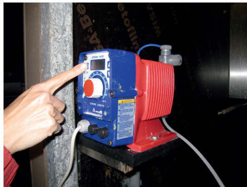
Figure 2.17 Dosage pump for pH regulation by preset dosing of NaOH. The pump can be connected to a pH sensor for fully automatic regulation of pH level.
