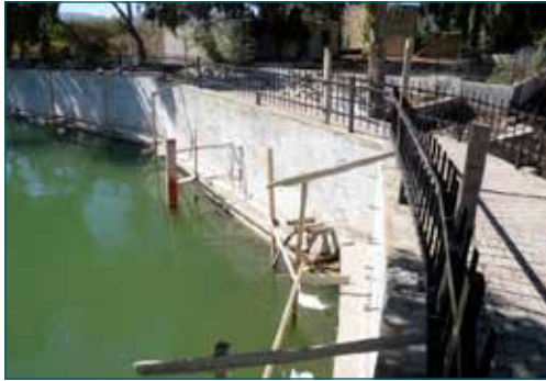
Figure 12: Results of Dardara pond rehabilitation
