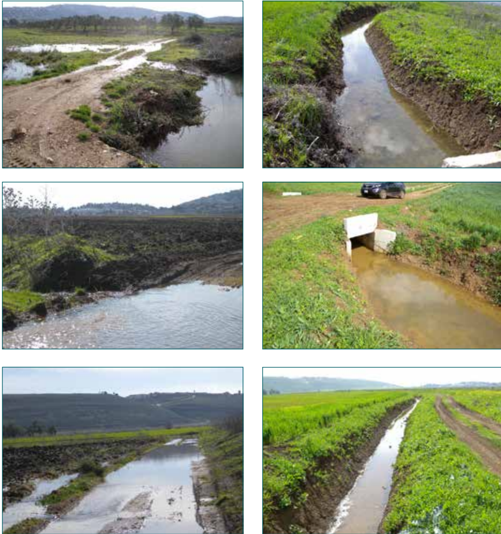
Figure 11: Pictures showing drainage before (left) and after (right) the intervention
