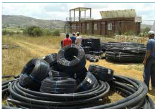
Figure 13: Delivery of the equipment
