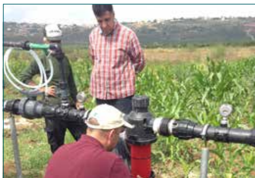
Figure 15: Inspection and operating
