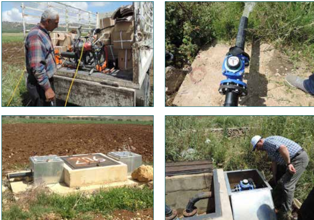
Figure 9: Figures showing the installation of flowmeters
