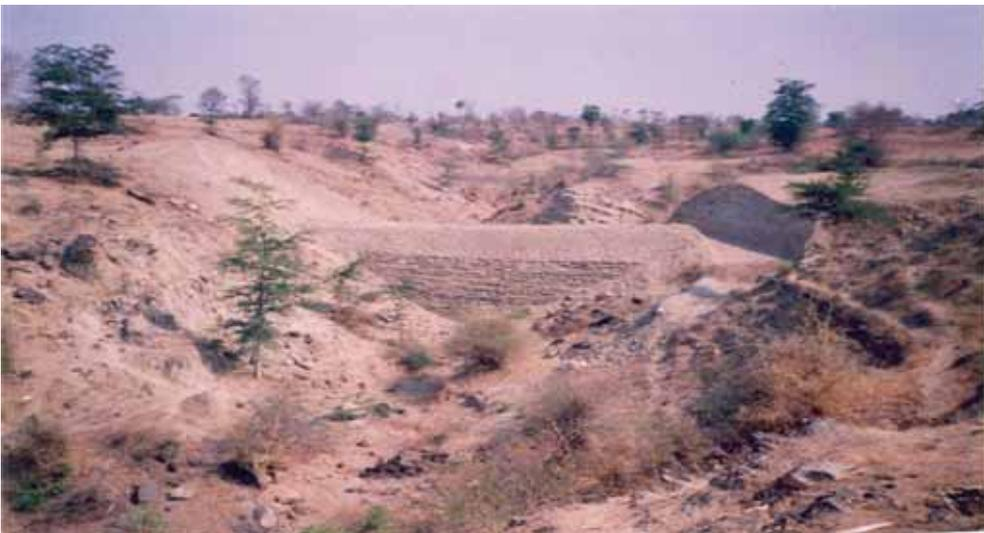
**Figure 4.** Sediment storage dam in the dry zone (for soil protection)
