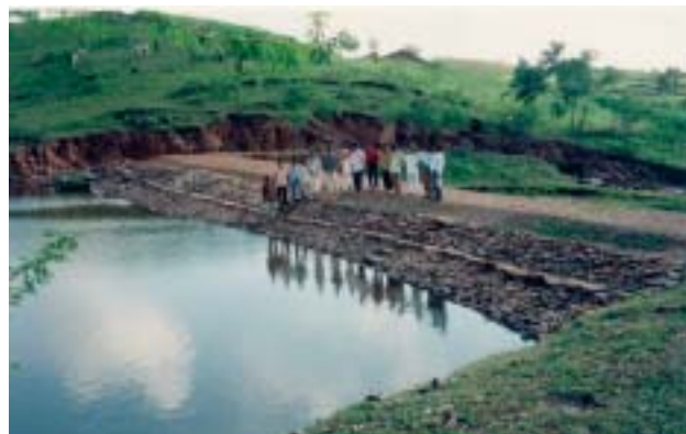
PLATE 21 Detention of sediment-laden runoff by a dam wall has been used to provide limited areas of flat cropland (here under rice); this may have been one of the purposes of the dam. Sharam, India [T.F. Shaxson]
