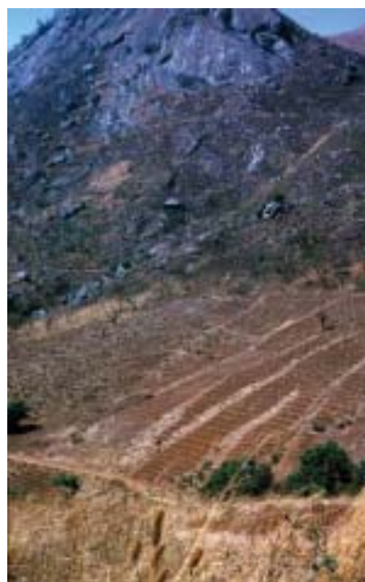
PLATE 47 Example of the effects of excessive rainwater breaching contour ridges at low points resulting in loss of rainwater by runoff and severe soil erosion – Mua, Malawi [T.F. Shaxson]
