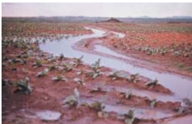
PLATE 51 A broad-based earth bund set on the true contour can cause local waterlogging if the collected runoff cannot soak in or flow away. Kasungu, Malawi [T.R. Jackson]
