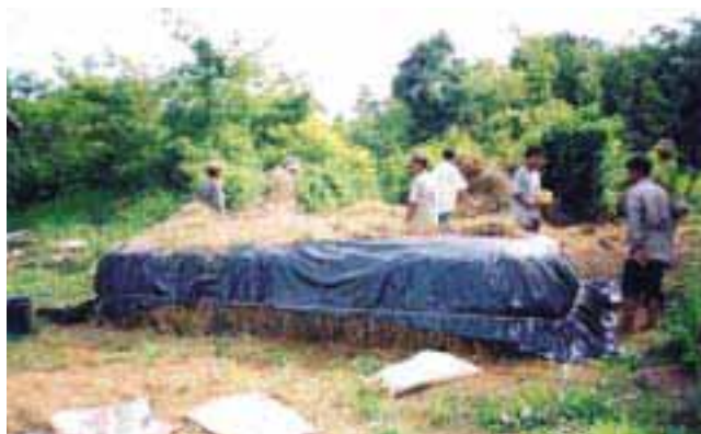
PLATE 5 The pile is covered with a plastic sheet after attaining the desired height [Singvilay (TCP/LAO/2901), Lao PDR]
