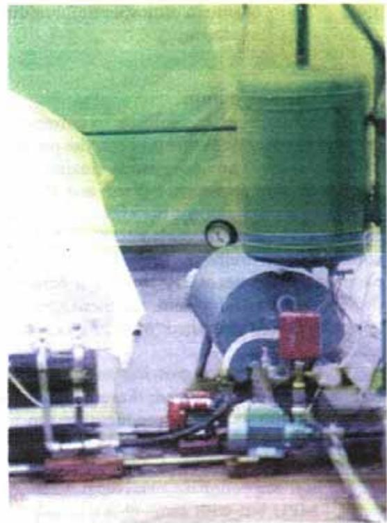
*Plate 2. Pressure tank for mist spray system and boiler, and circ. water pump heating system*
