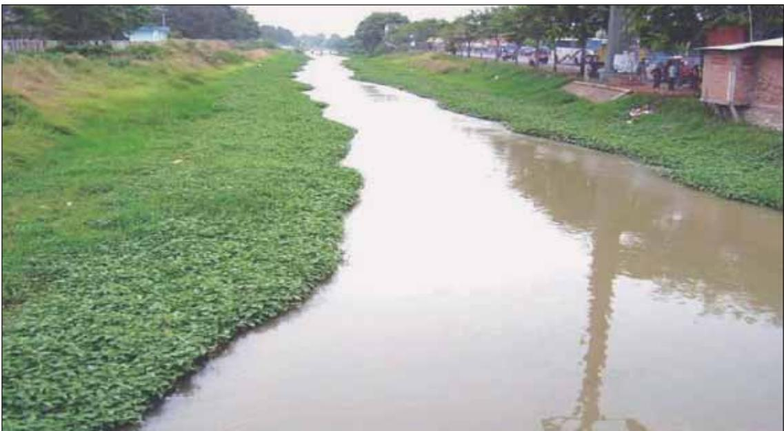
**Figure 5. Weeds in unlined canal**
