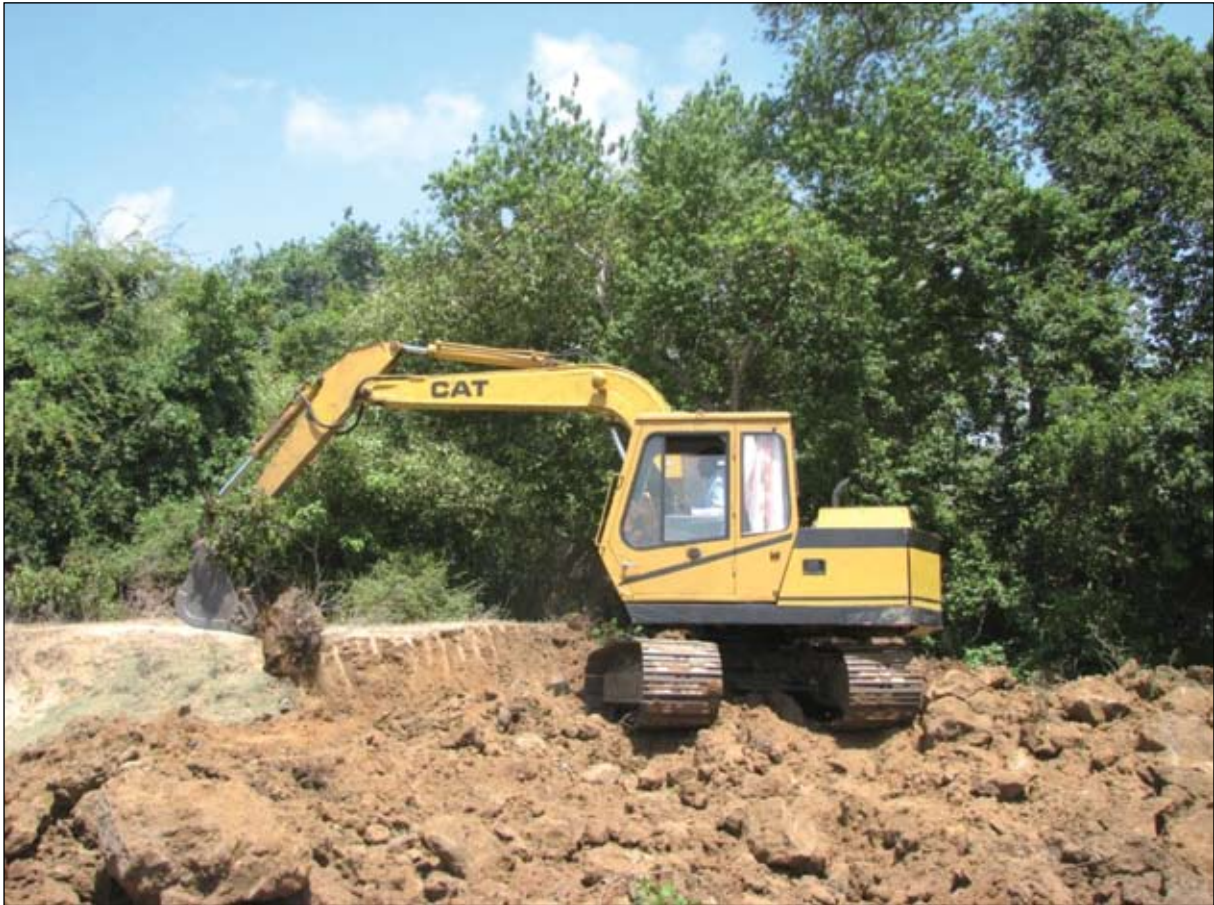
Figure 77. Clear-felling mangroves in the Puttalam Lagoon area (© Dilup Chandranimal)
