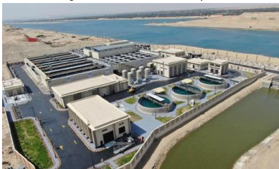
Figure 3.2 Al Mahsama treatment plant
