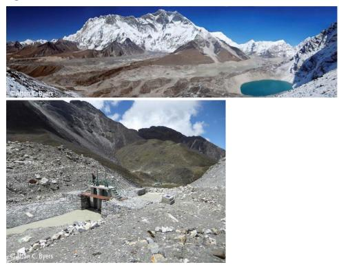
(Top) Imja glacial lake, which is a potential hazard to downstream communities and infrastructure in the event of a glacial lake outburst flood. (Bottom) Draining Imja glacial lake in 2016 by constructing an outlet canal and control gate.
