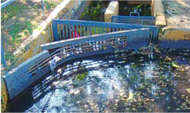
Solid waste trap at packing plant. Photo Miguel Vallejo
