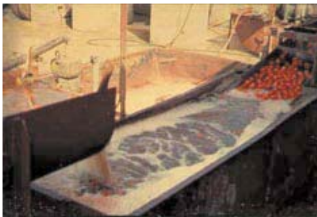
Figure 16.3: Tomato fluming operation, circa 1960.
