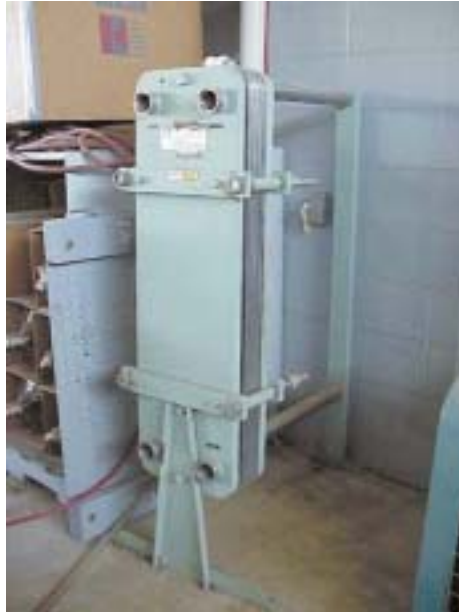
Figure 8.5: Plate heat exchanger.
