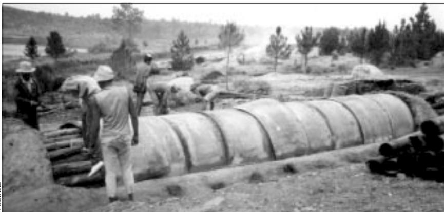
*A semi-permanent low-cost "Subri-fosse" type metal kiln in Madagascar was designed to carbonize offcuts from sawmilling*
