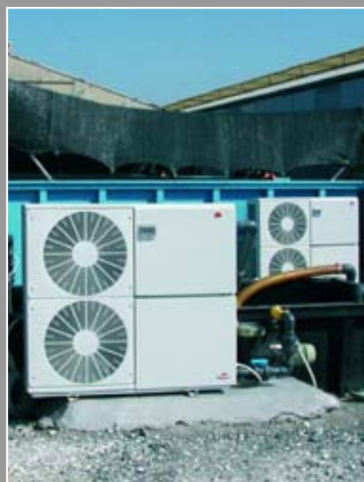
Fig 82 - Heat pumps
