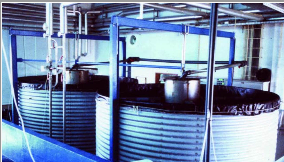
Fig. 66 - Trickling filter
