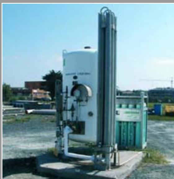
Fig. 73 - Liquid oxygen reservoir and oxygen bottles
