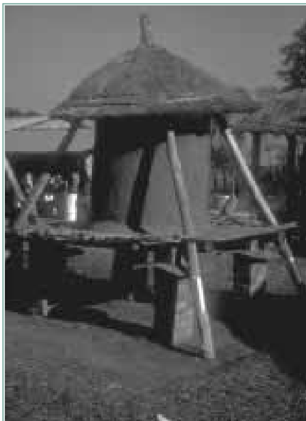
FIGURE 5 An improved grain-storage silo made from local materials in Malawi.
