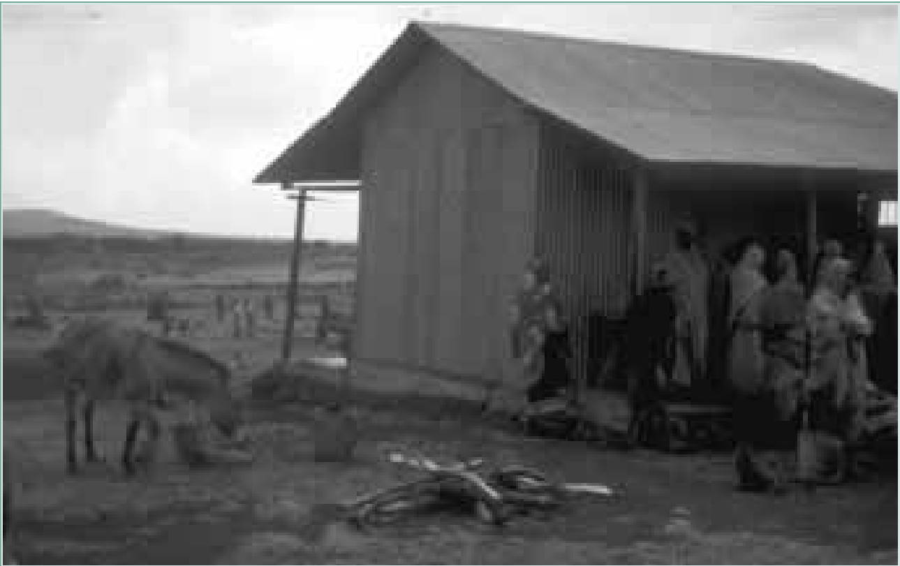
FIGURE 17 Galvanized-steel building for village hammer mill in Kenya.
