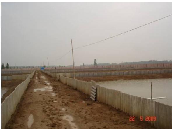
Photo 3-5-1 Concrete wall of fish pond in Caolou Village
