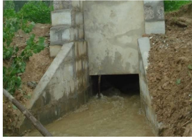
Photo 3-3-2: Outflow of the Culvert (photo by Wang Yanguai)
