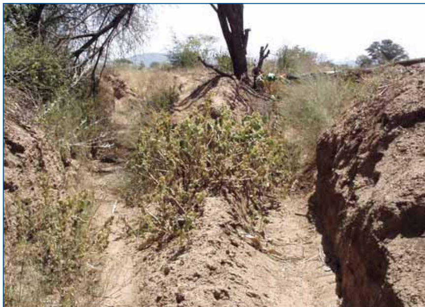
Flow division in a flood canal, Yanda-Faro, Konso, Ethiopia
