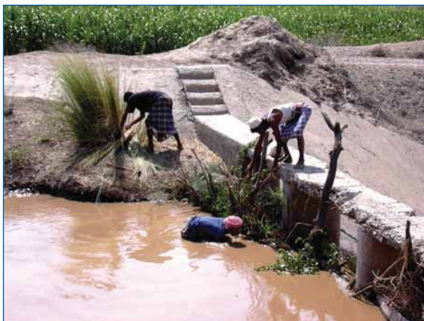
FIGURE 8.3 Farmers using brushwood to head up the flow in a canal. Wadi Tuban, Yemen
