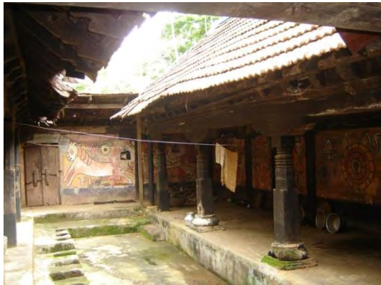
Figure 11: View of the staircase
