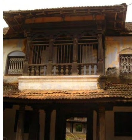
Figure 2: View of the balcony
