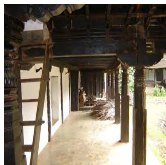
Figure 14 View of the wooden ceiling
