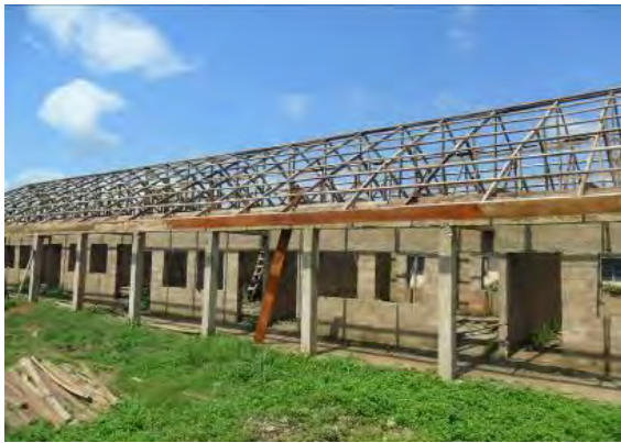
Plate 1 a: wood in roof of classroom construction
