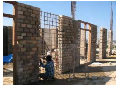
Figure 15: Bamboo Crete wall
