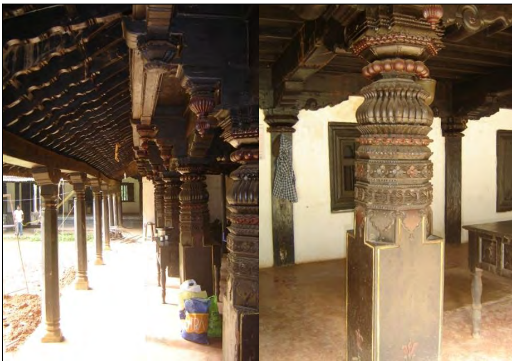
Ornamental Wooden Column and beams
