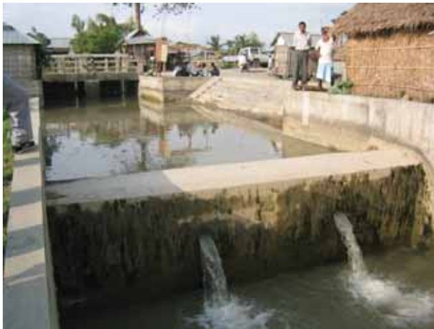
Plate 3 Example of wrongly designed measurement crest at the headworks of a secondary canal along the CMC raising the water level and leading to excessive sensitivity of the offtake.
