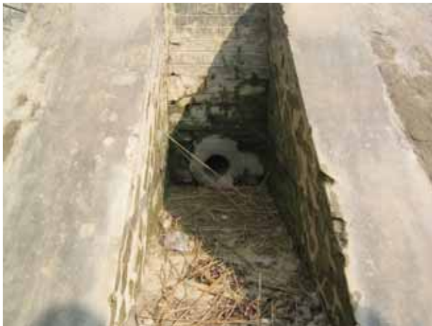
Plate 9 Ungated reduced diameter pipe outlet in the NIS.
