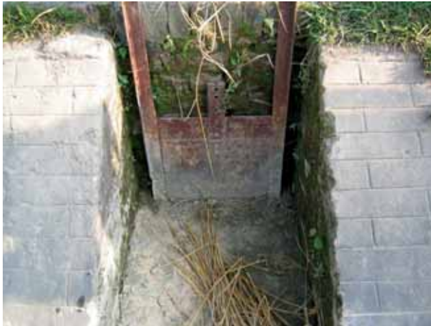
Plate 8 A few of the remaining original tertiary canal control gates in the NIS.
