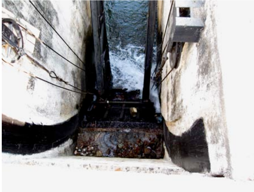
Plate 6. Servicing drainage escape ditch: non repaired leakage on an escape gate to served population along the drainage (Y Jonction Naryanpur canal)
