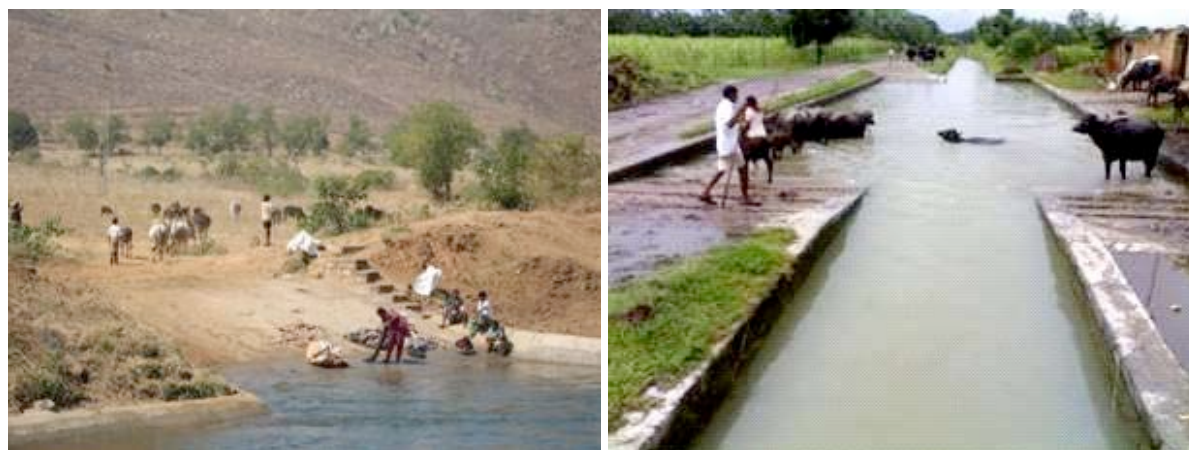
Plate 16 Examples of ramp easing water access for animals (Bhadra Karnataka-left; Main Ganga UP -right) .
