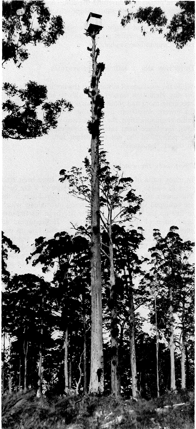
38. Fire-tower on the "Gloucester tree," a 60-m-high E. diversicolor , at Pemberton, Western Australia (photo taken in about 1955) Forests Department, Western Australia
