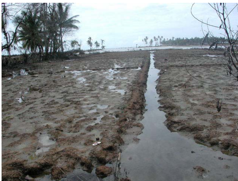
West Aceh: Due to land subsidence the drainage system is now influenced by the higher sea water level and drainage capacity is reduced.
