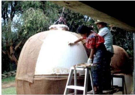
figure 7.2: Hand lay up of jute on a PVC balloon
