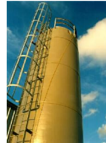
Silo de stockage de coulis (40 kWh m -3 ) Ice slurry storage silo
