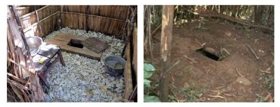
Composting Toilet and Septic system – In a composting toilet, the facility is built above the composting bin. This makes it easier to remove the bin so that it can be emptied and used as plant fertilizer. In a septic system, the waste uses water to move the waste from a flush toilet to a special tank that holds the waste until it can be pumped using specialized equipment.
