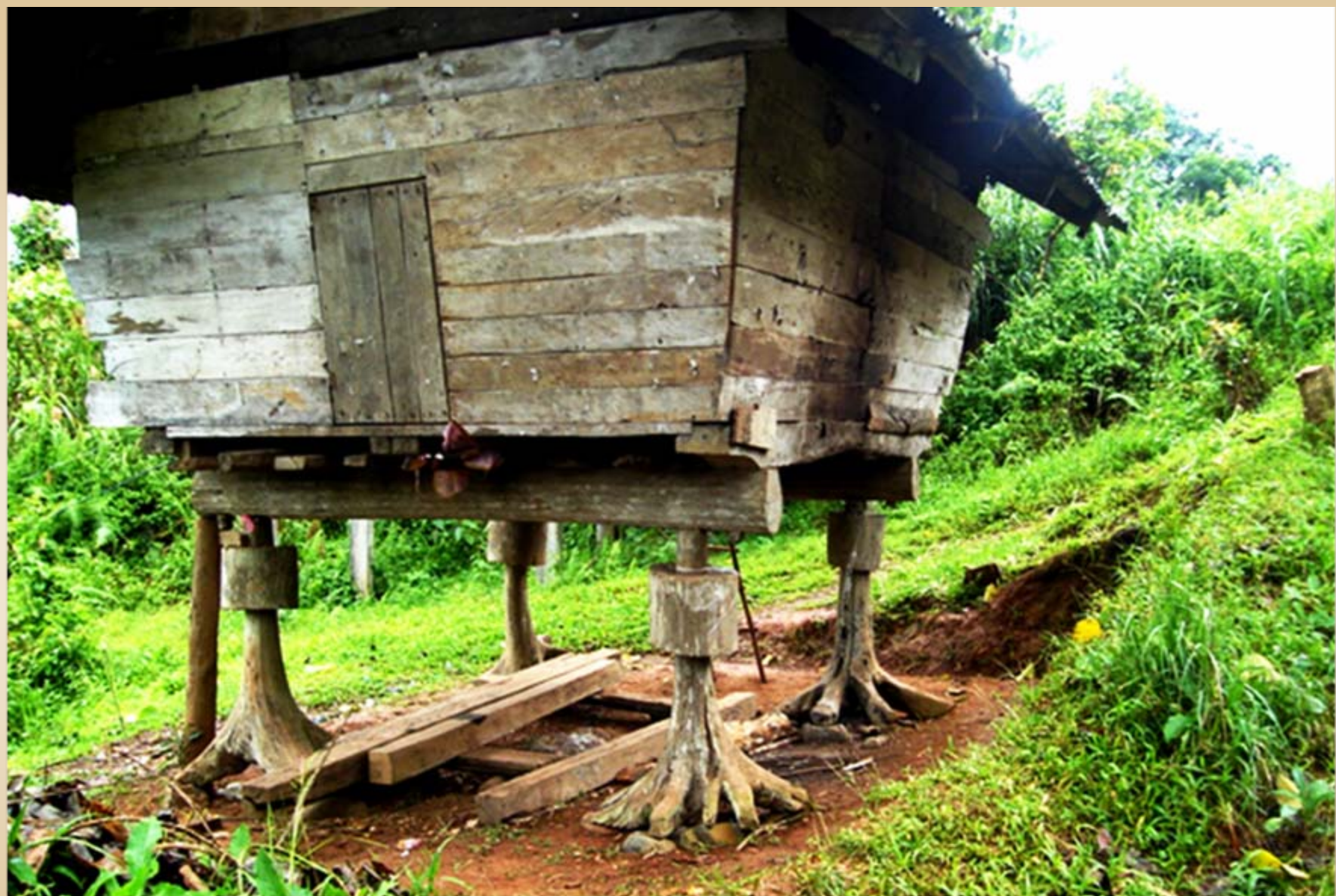
The traditional rice granary of the Ifugao's. Note the posts made of tree stumps sourced from the Muyongs.
