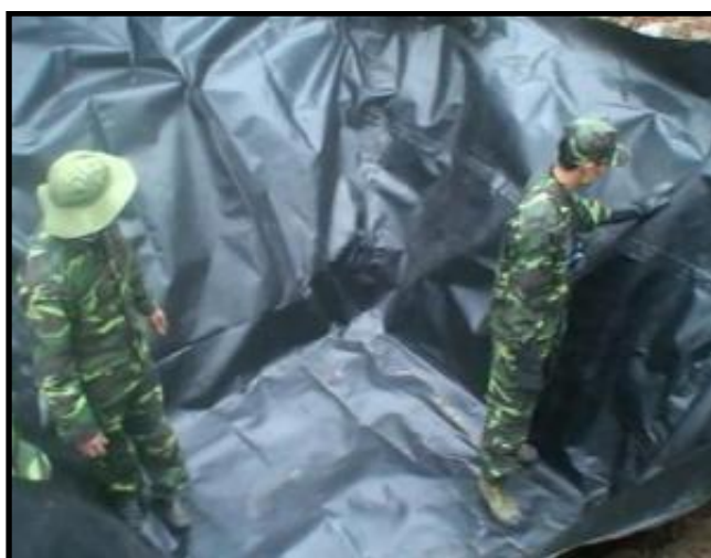
Photo 1: Burial pit lined with impermeable plastic sheet.
