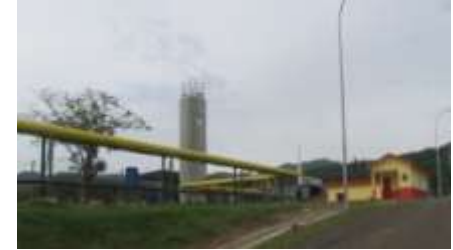
BIOGAS CAPTURED PIPING TO BIOSCRUBBER
