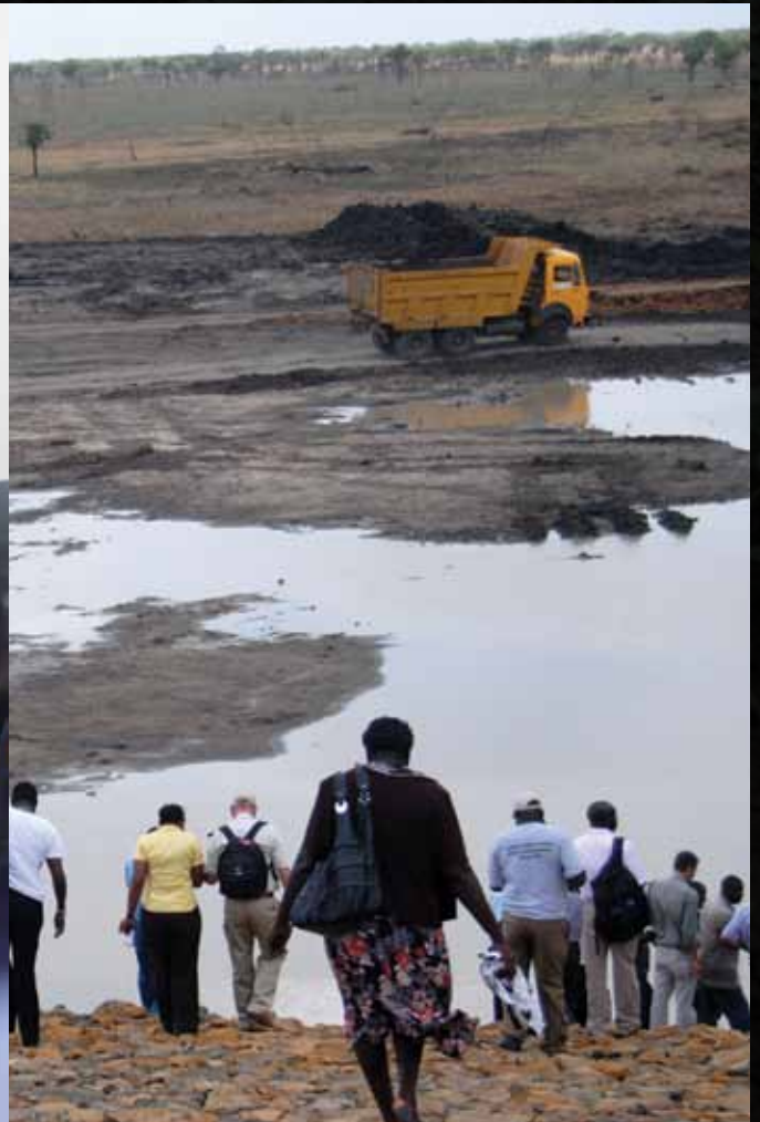
▲ The Government is constructing a dam in Moroto
