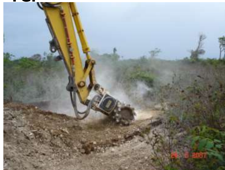
Machine used to pulverize rocks in the Cayman islands
