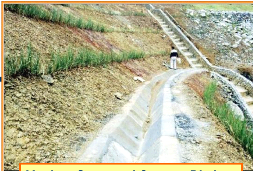
Vertiver Grass and Contour Ditches
