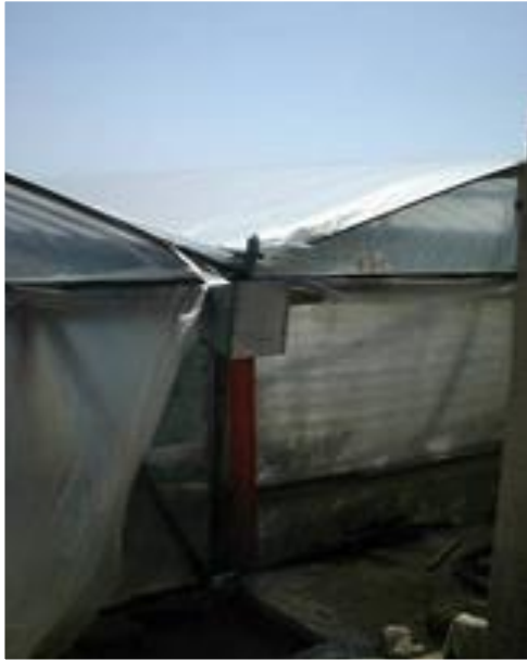
Rain water recovery from permanent greenhouse
