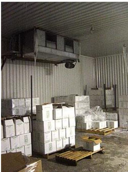
Figure 27 Refrigeration chamber to maintain avocados at 3 to 7 °C.
