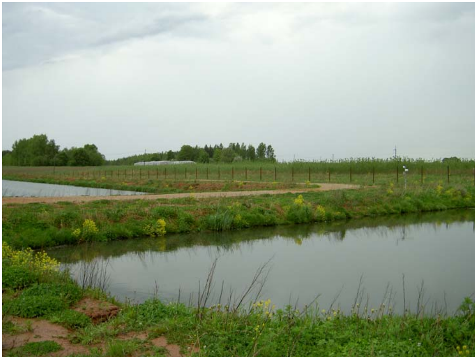
Kambja domestic sewage facultative ponds with willow plantation in background
