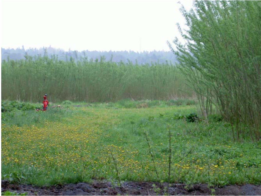
Wastewater valve within the Enköping willow plantation
