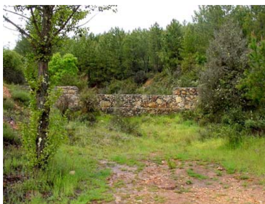
Fig 3. Gavion masonry stabilisation dam.
