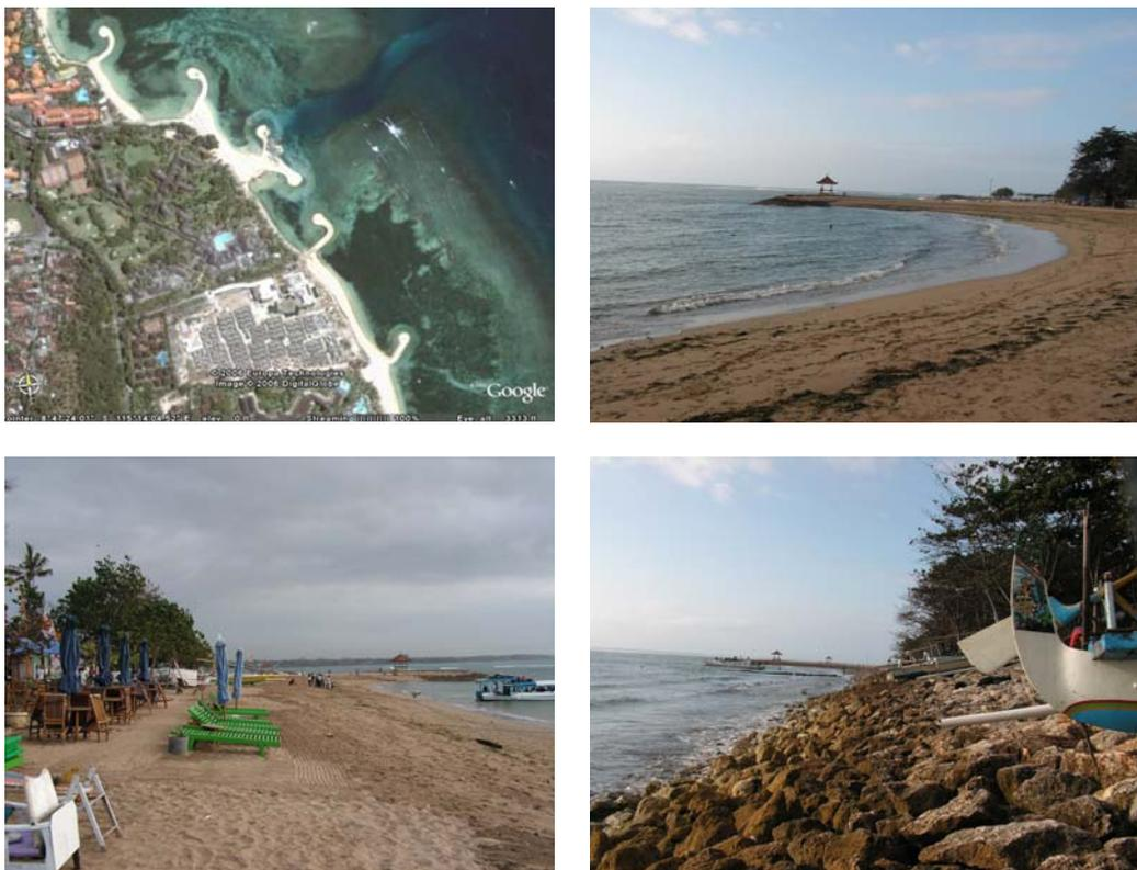
**Plate 4.1 Different types of coastal protection structures in Tanjong Benoa and Sanur Bali for protecting the valuable tourism base. Clockwise: Satellite images of the offshore breakwater and artificial headland, groynes and beach nourishment (Google maps); headland and beach nourishment with coconuts; loc cit *waru* trees; revetment protection using limestone in combination with *waru* trees (note the dangerous placing of the boats)**
