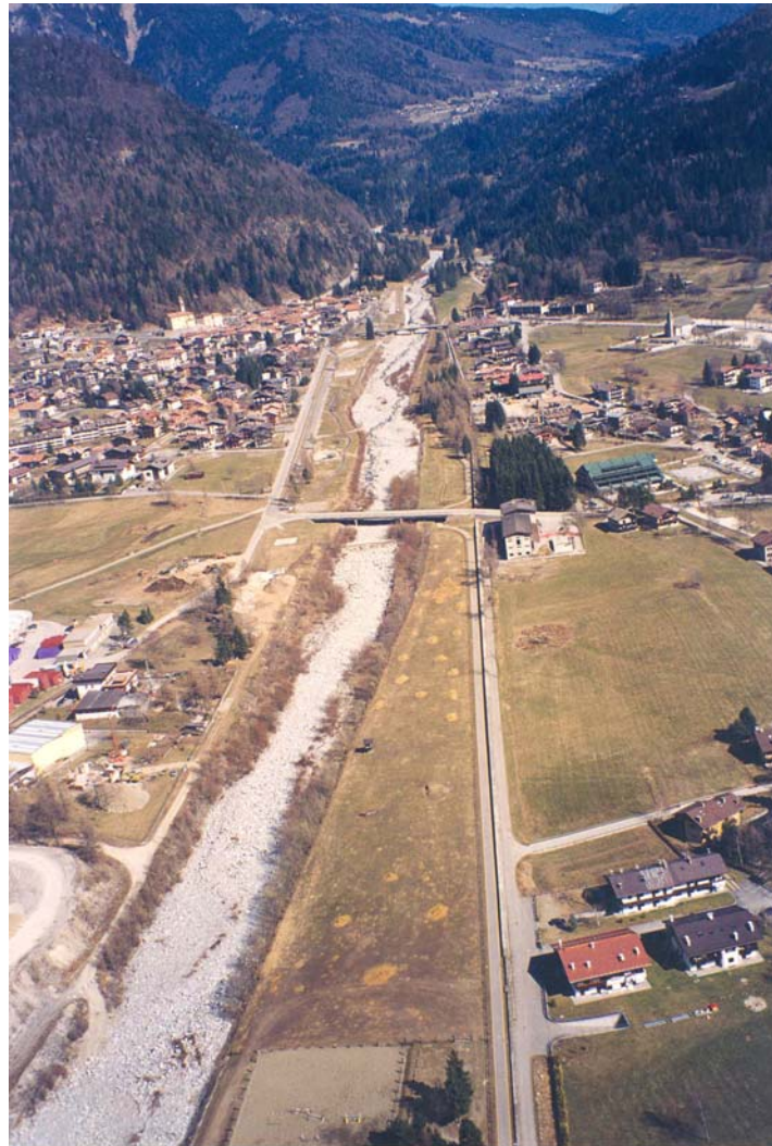
The Sarca torrent control in the Municipality of Pinzolo, Val Rendena, Italy (Photo: Servizio Sistemazione Montana, Autonomous Province of Trento, Italy, 2004)
